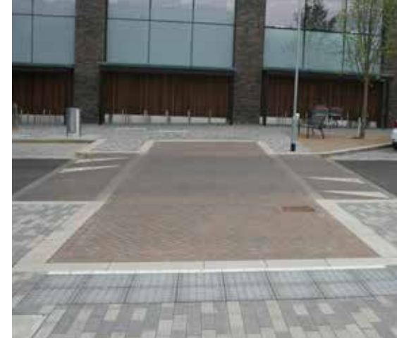
RAISED TABLES MARK VILLAGE ENTRANCES & 20 MPH ZONE
